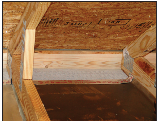
With roof edge flashing, fewer embers enter the attic area. Photo by Institute for Business and Safety Research Center.
