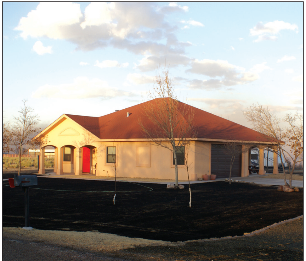
Firewise construction and landscaping helped protect this home from wildfire.
